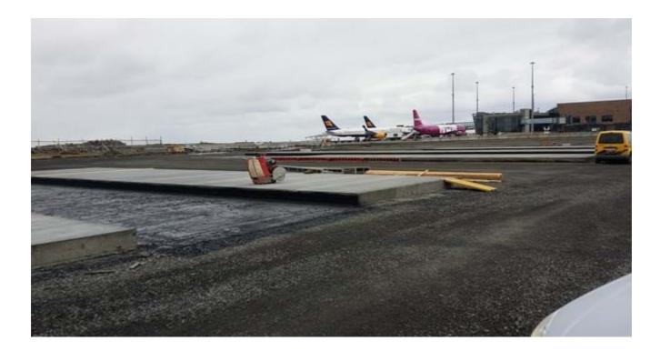
IAV's scope of work was excavation, and filling under the new apron, sand traps, oil separators and foundations of light towers.
